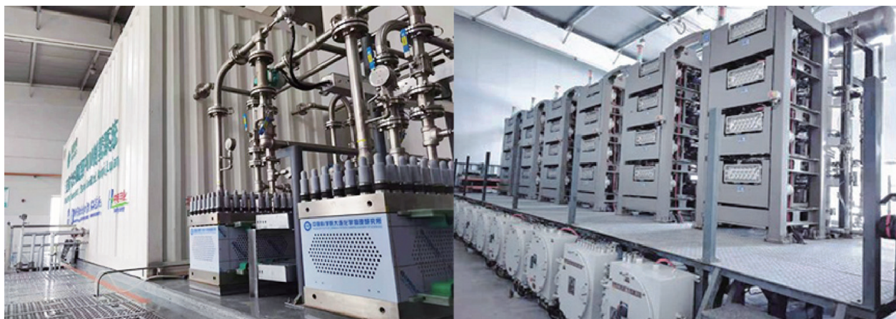
The megawatt-level proton exchange membrane (PEM) water electrolysis hydrogen production system (left) and the megawatt-level hydrogen proton exchange membrane fuel cell power generation system (right).
