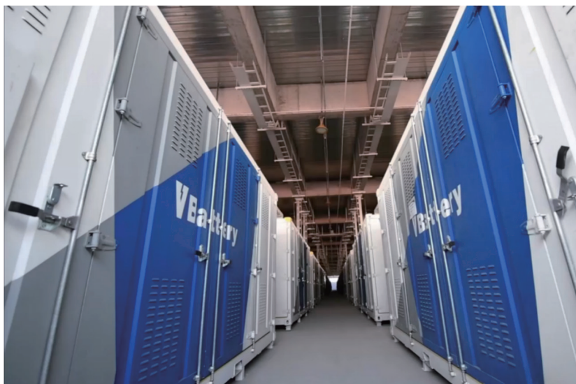
A 100MW/400MWh vanadium flow battery energy storage power station for peak shaving that reduces strain on the grid.
